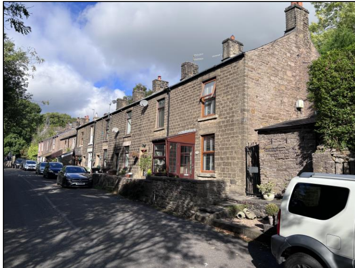
Figure 3: Front Elevations looking from the west
