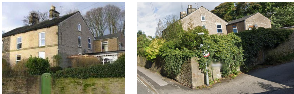
Fig.2 Image of No. 36 accessed from Chapel Road and 36a accessed from Rock Bank. Image taken from sales particulars of the most recent sale of 36 Chapel Road in 2007.
