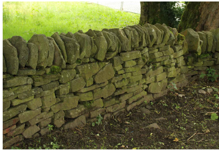
Reference: Existing Dry Stone Wall on Site
