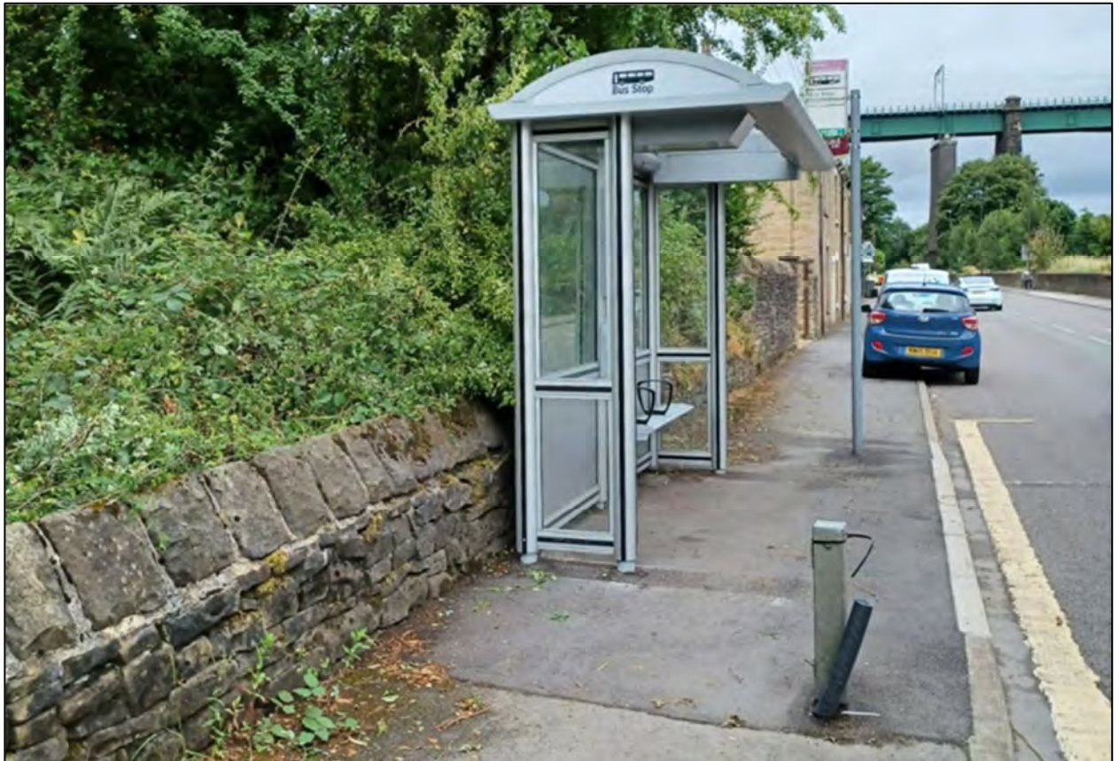
Figure 3.1 – Existing Bus Stop
