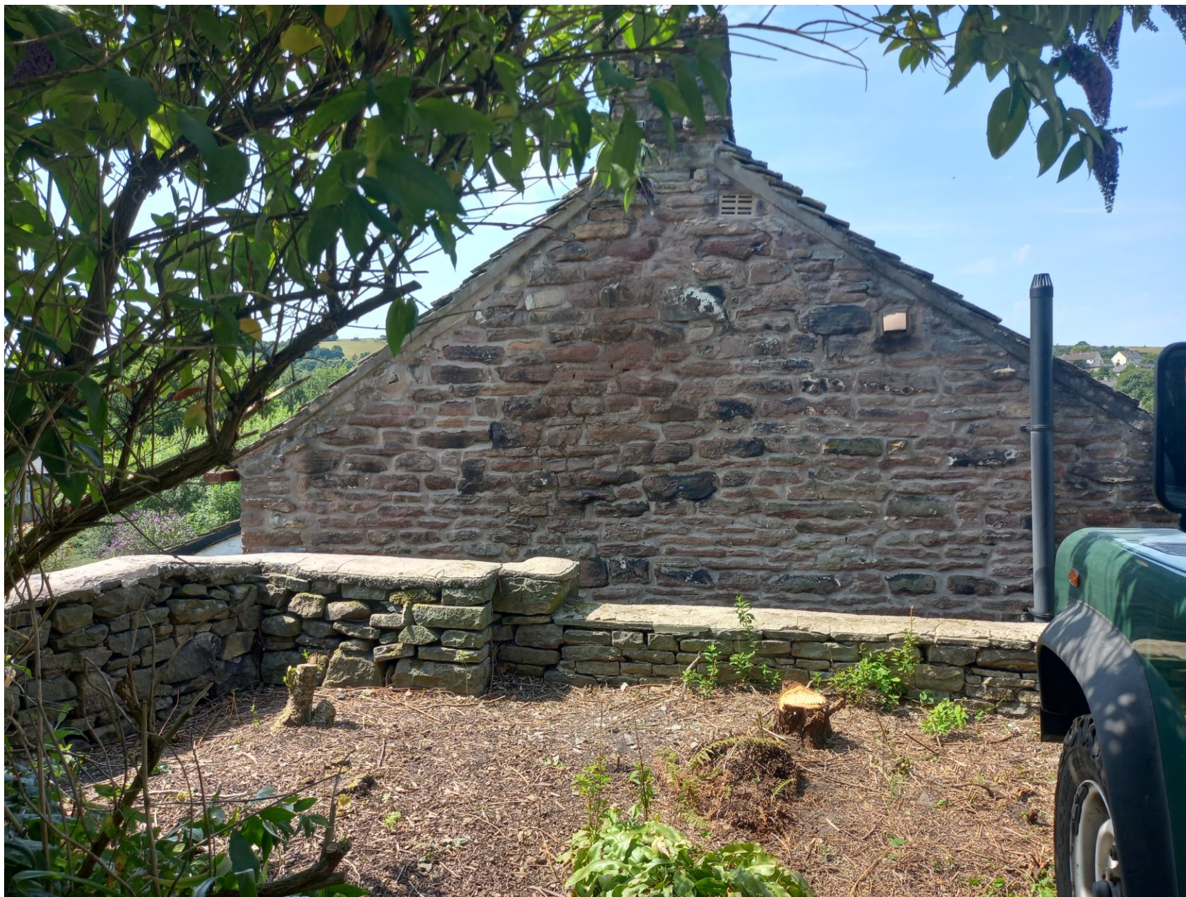
GABLE WALL OF 2, BINGS ROAD, WHALLEY BRIDGE.
