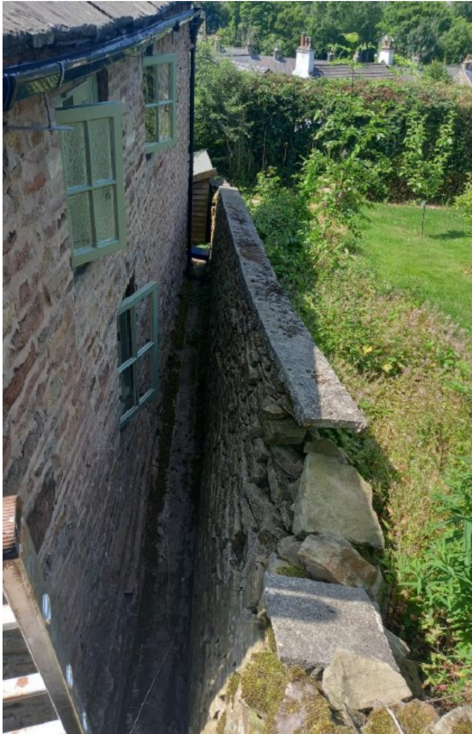
Figure 5: Proximity of the Existing Retaining Walls
