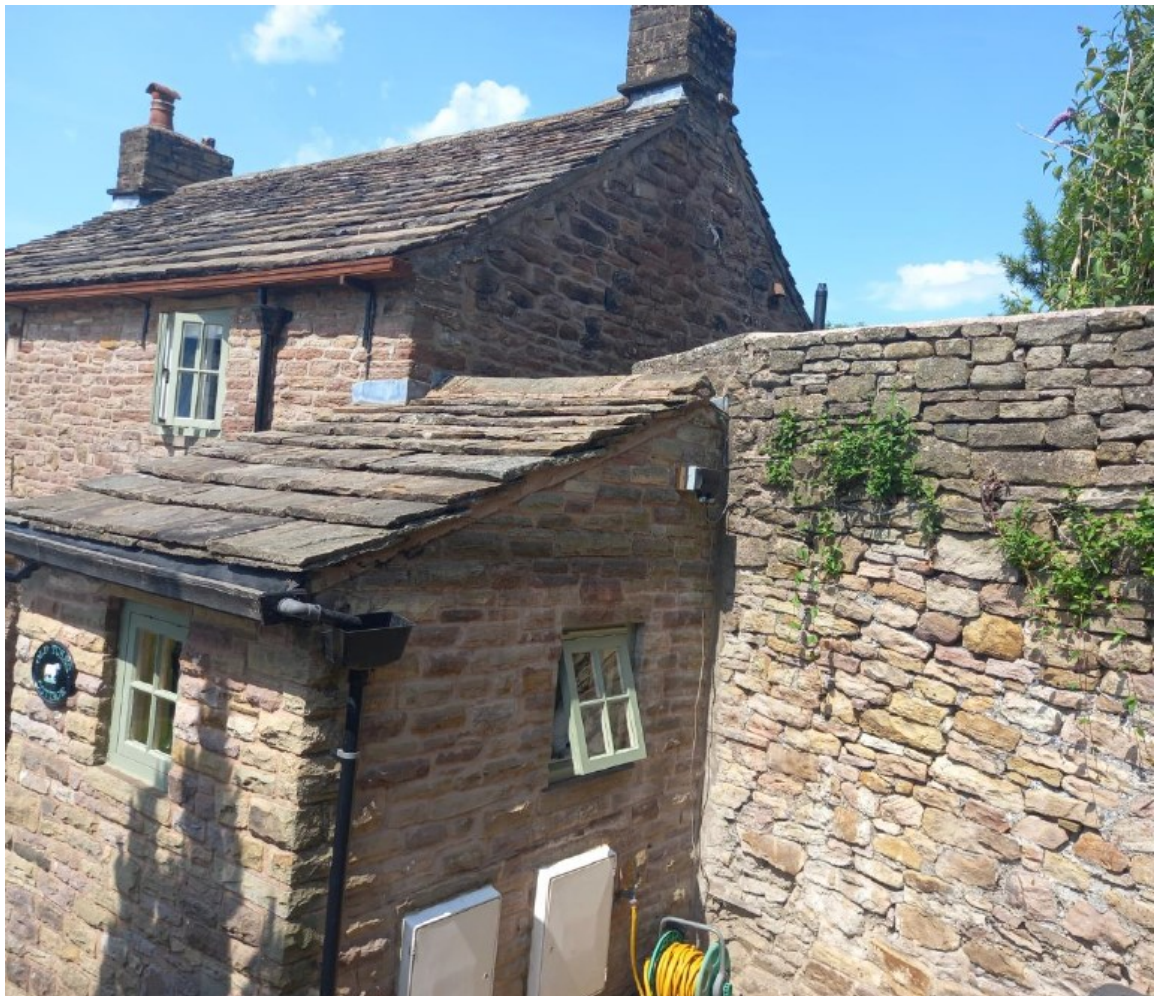
Figure 4: The Existing Side Extension
