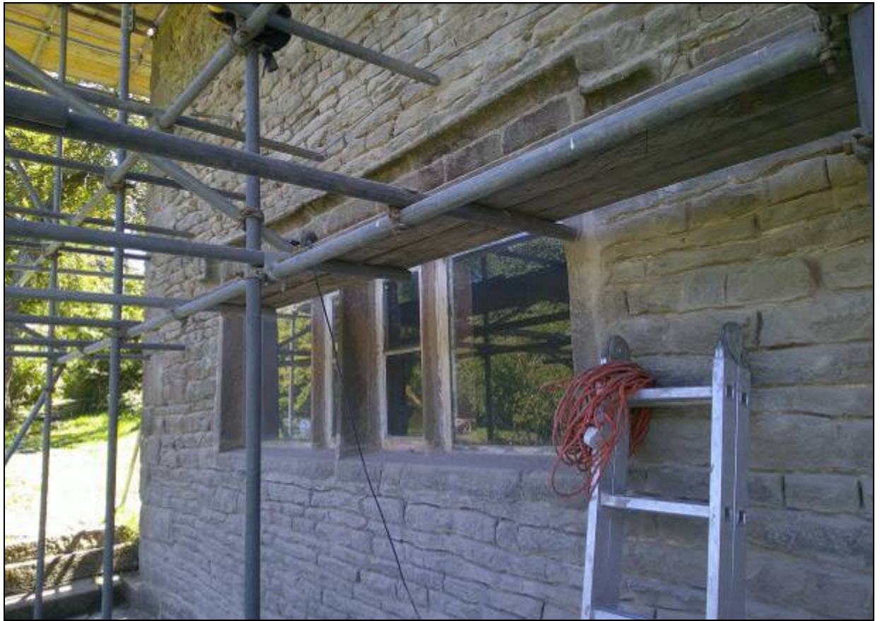
6. The originally six-light window on the rear elevation
