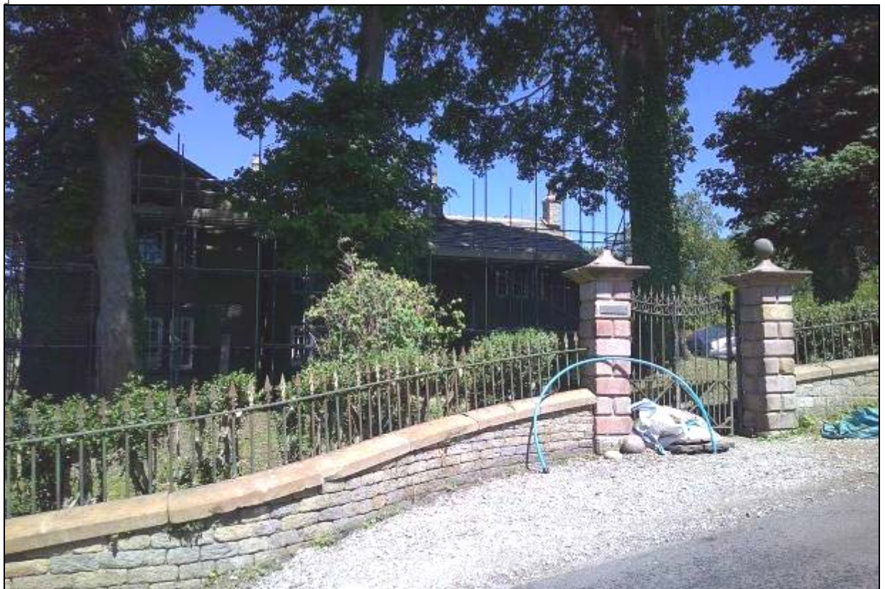
2. Gatepiers mark the original main entrance to the site
