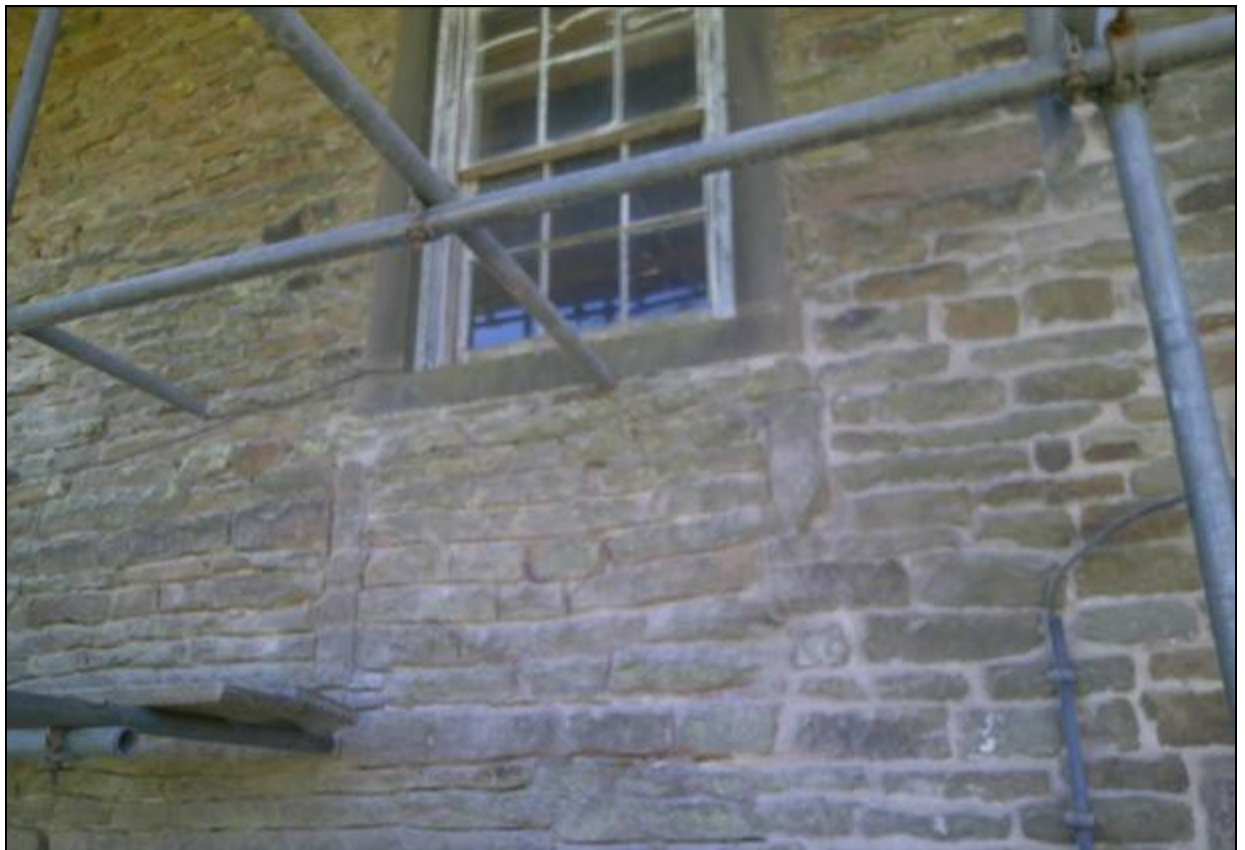
7. Sash window replacing original stairlight, now blocked beneath
