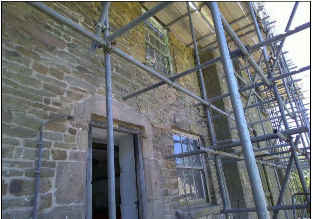
8. Mid-late 19 th century six-pane sash right of door, 16-pane sash above
