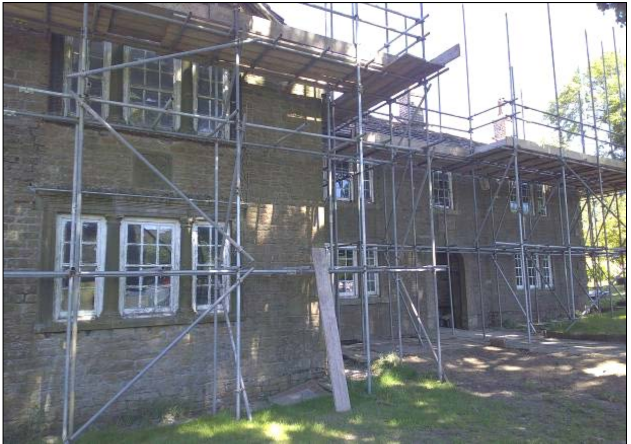
3. Front elevation of the building: windows are early-mid 20 th century
