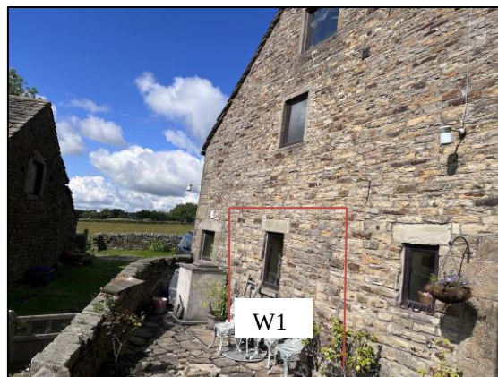
Figure 12: W1 (external) showing the approximate extent of wall removal outlined in red
