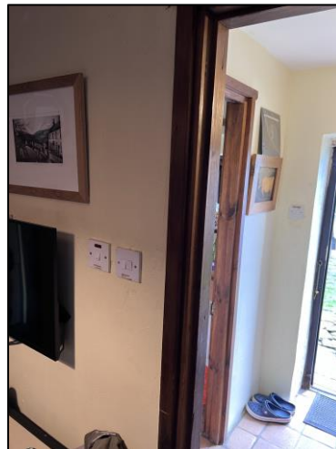
Figure 12: D2 and D3 internal door frames and stud partitions.
