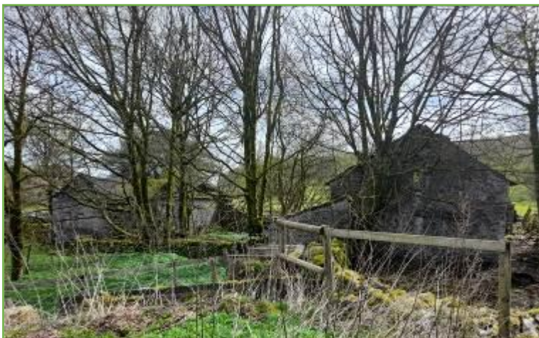
Picture 3: View showing 85 and 87 Green Lane and extent of tree cover
