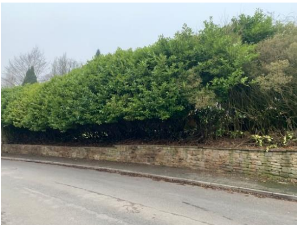
View from the front of No 6
