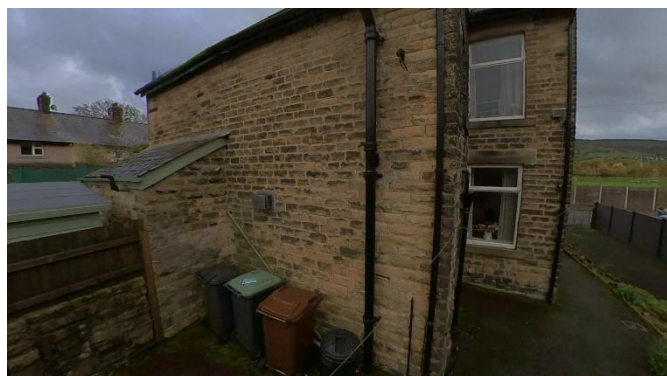
Existing Rear of 38 & 40 Spire Hollin
