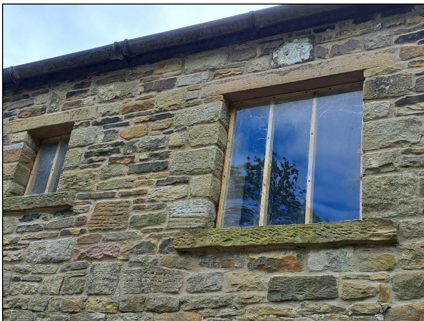
Photograph 2 showing the stone lintels
