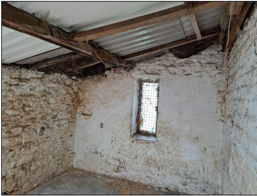
Photograph 7 showing the interior of the single-storey section
