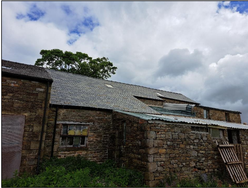
Photograph 3 showing pitched roof
