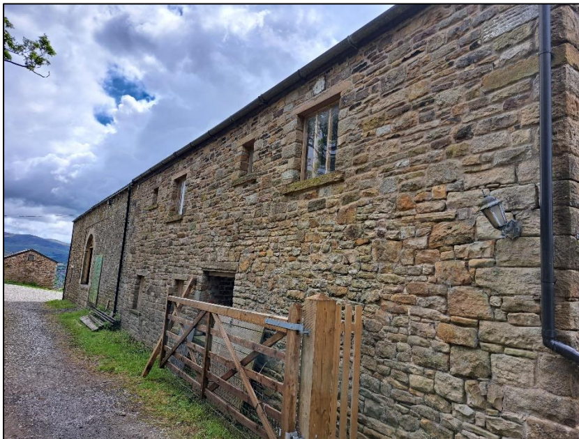
Photograph 4 showing the barn exterior
