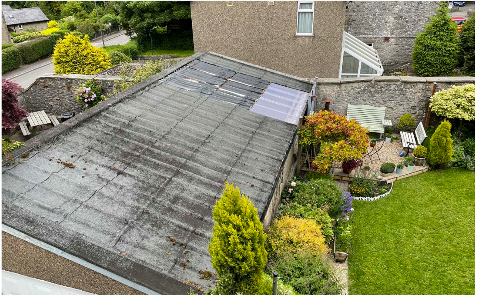
View of garage roof
