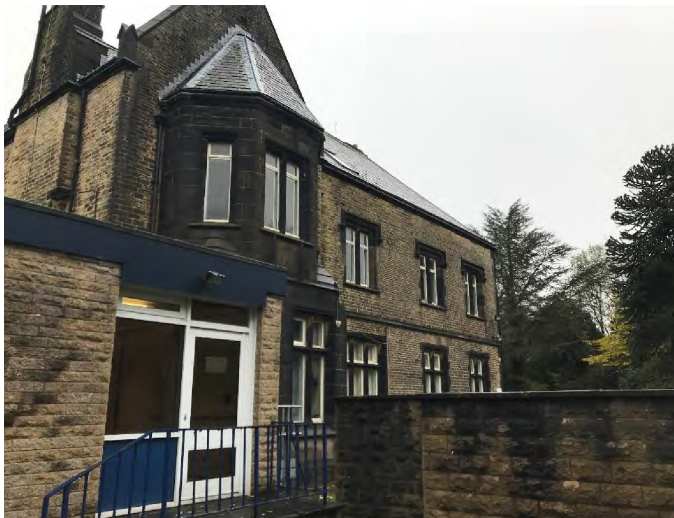
Front elevation facing southwest
