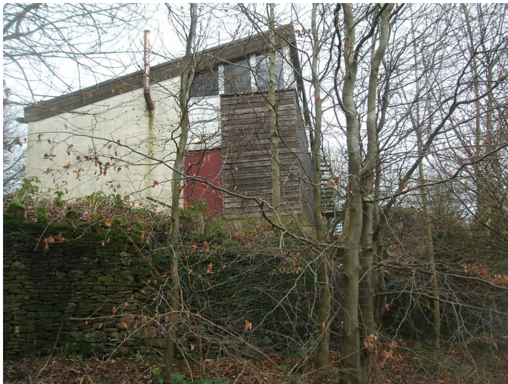
Figure 3: Approved location for semi-detached dwellings (viewed from the public footpath)
