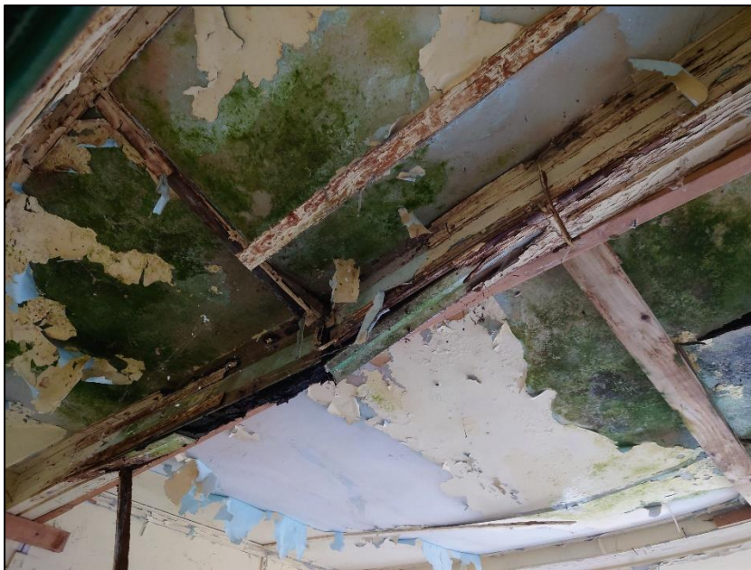
Photograph 5 showing the damaged roof joists
