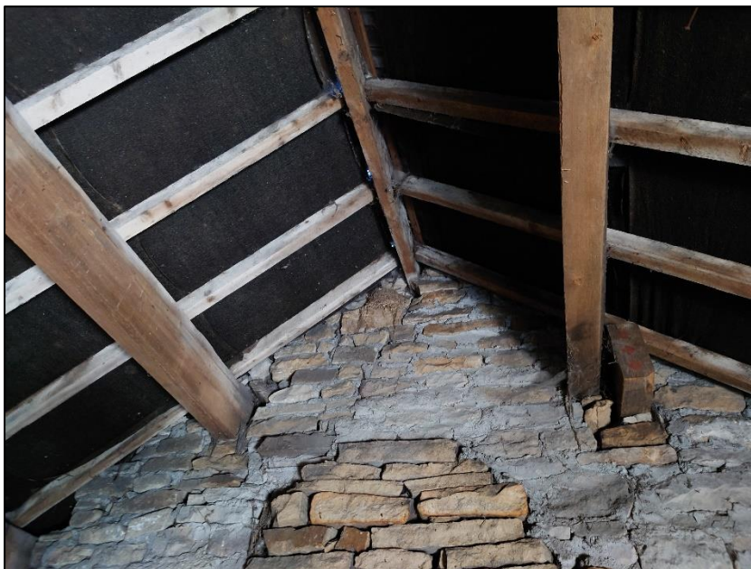
Photograph 10 showing the interior of Barn 2
