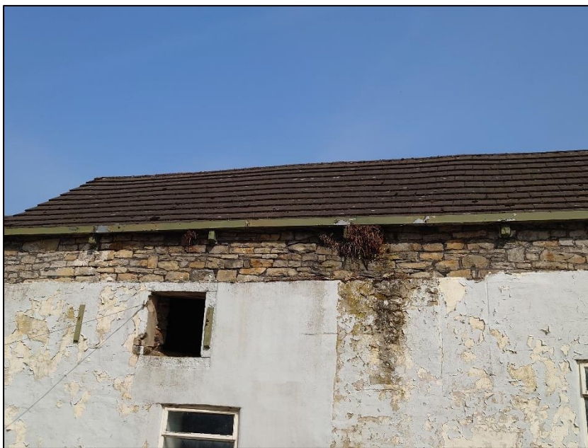
Photograph 3 showing the roof of the building
