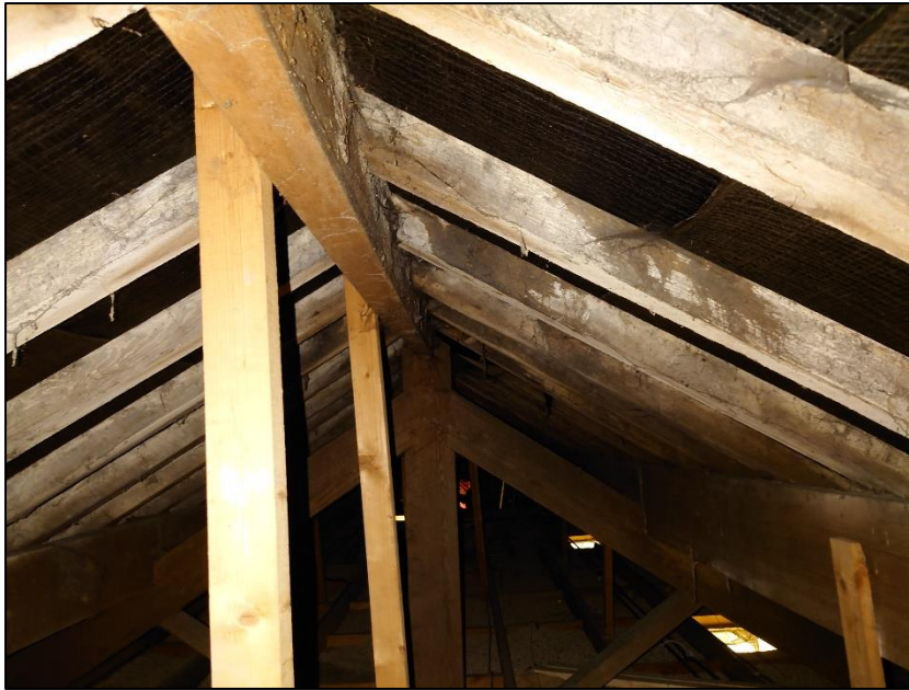
Photograph 11 showing the roof void of Barn 2
