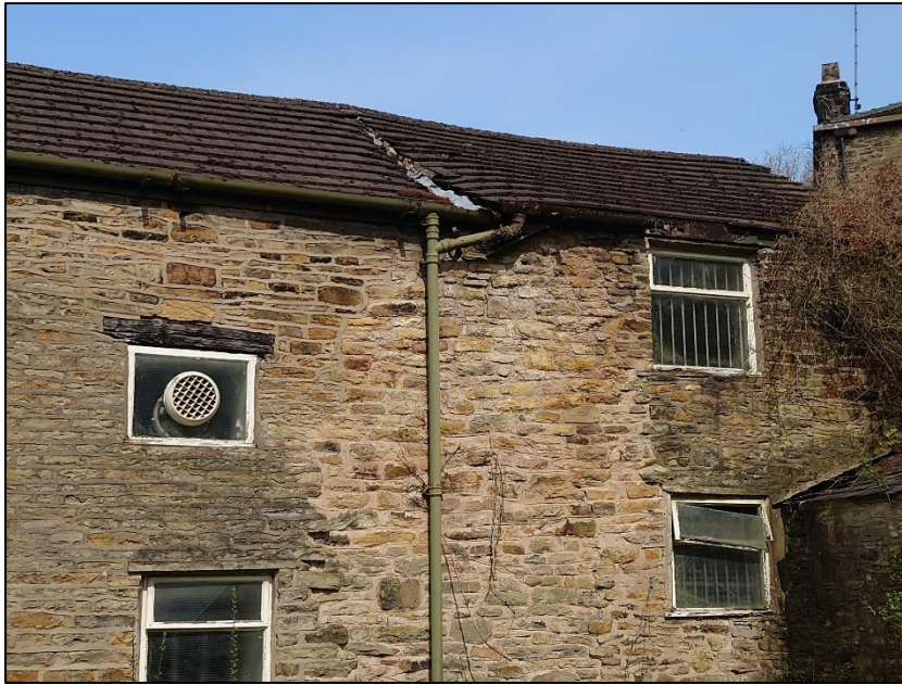
Photograph 9 showing the roof of the barn
