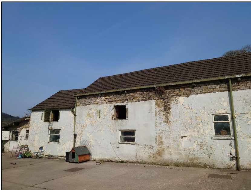
Photograph 1 showing the exterior of Barn 1
