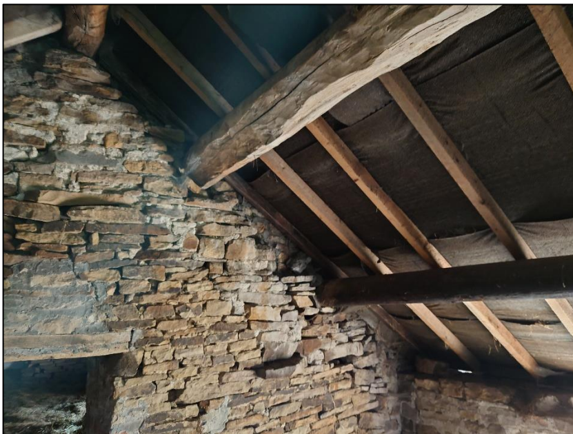
Photograph 4 showing the upper floor and internal stonework of Barn 1
