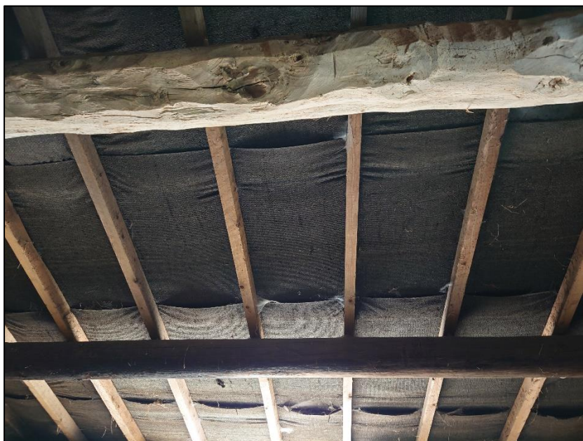
Photograph 5 showing the roof structure of Barn 1
