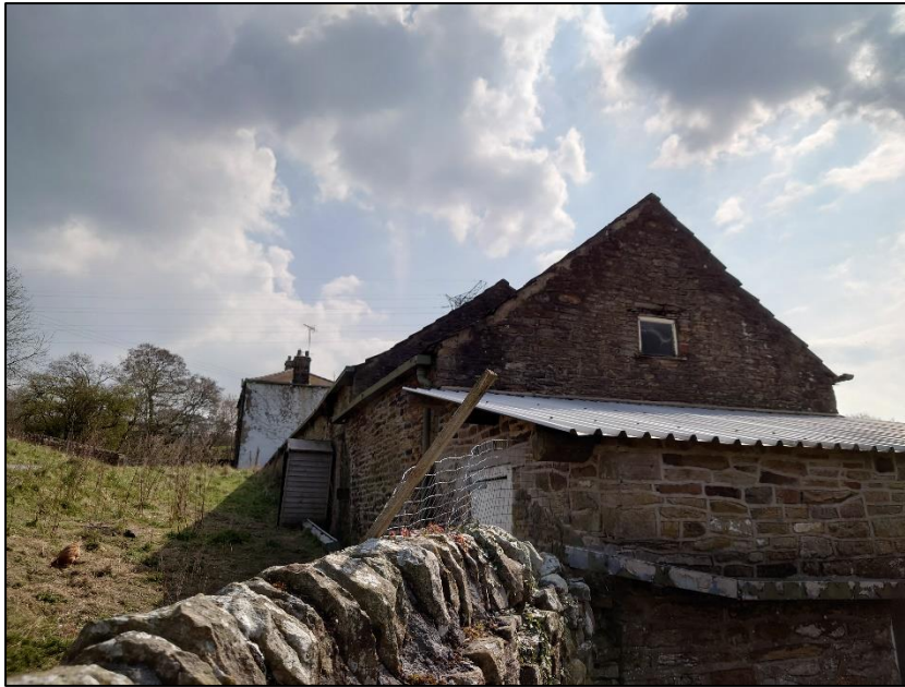
Photograph 2 showing the gable end of the building
