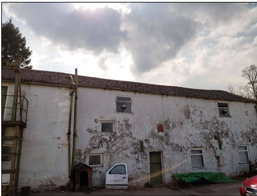
Photograph 8 showing the exterior of the barn
