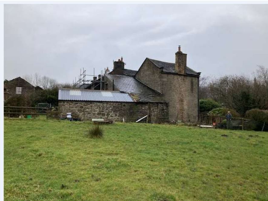
Above: View to western elevation from nearby Public Right of Way
