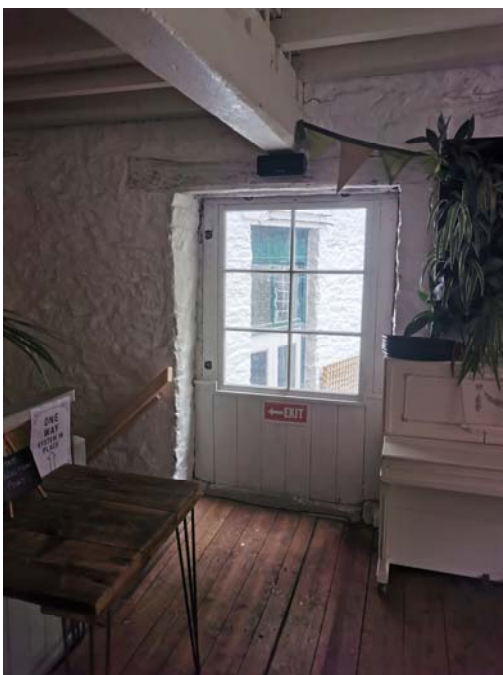
Left - WG01 Previous door opening with non original timber window infill. WG02 Below
