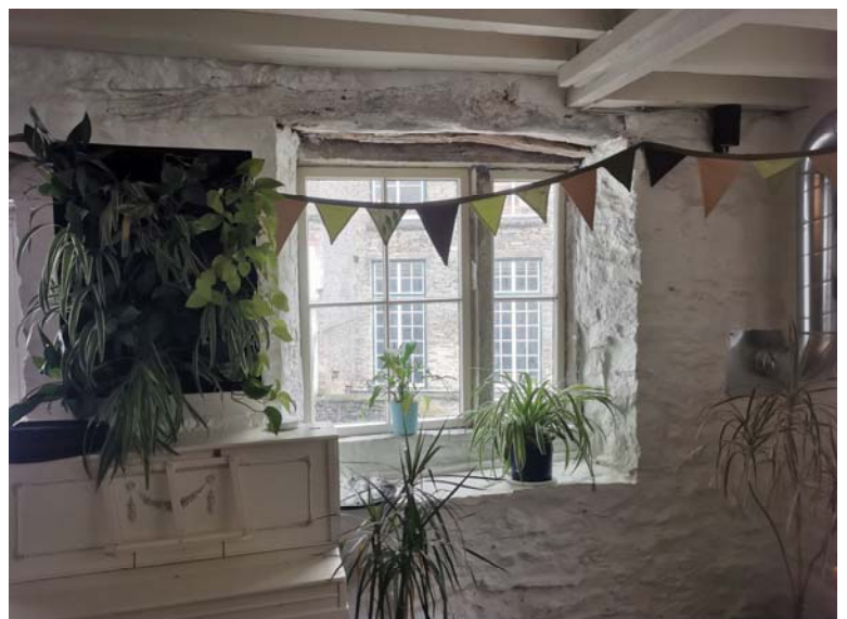
Left - WG01 Previous door opening with non original timber window infill. WG02 Below
