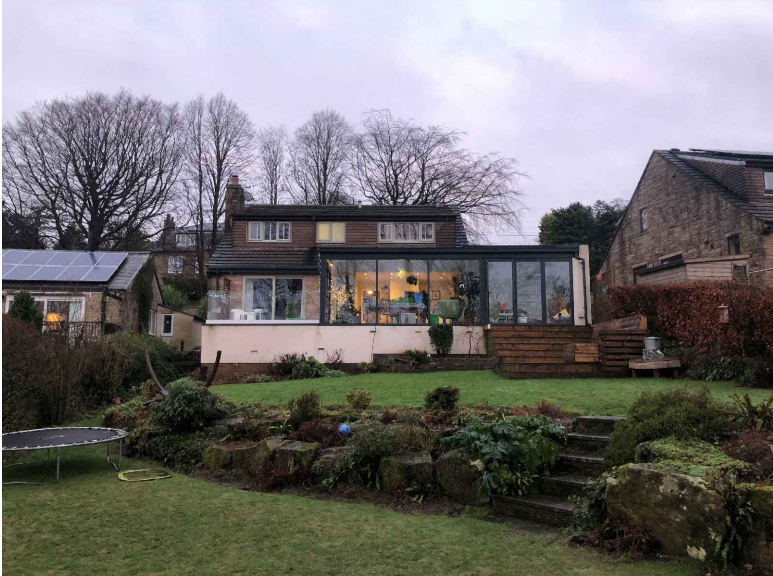
Existing south elevation - Rear Elevation Existing photos of property n.t.s
