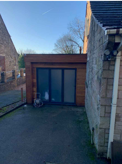
Existing north elevation - garage
