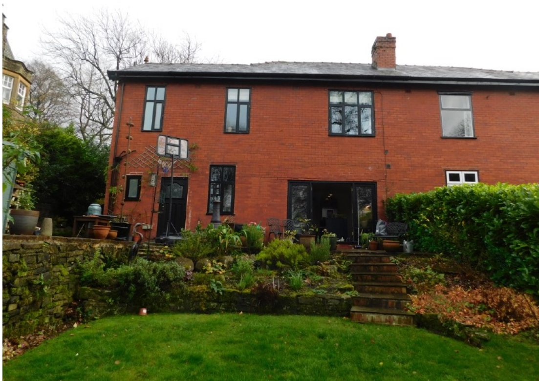
Rear Elevation - Danemoor, North Road
