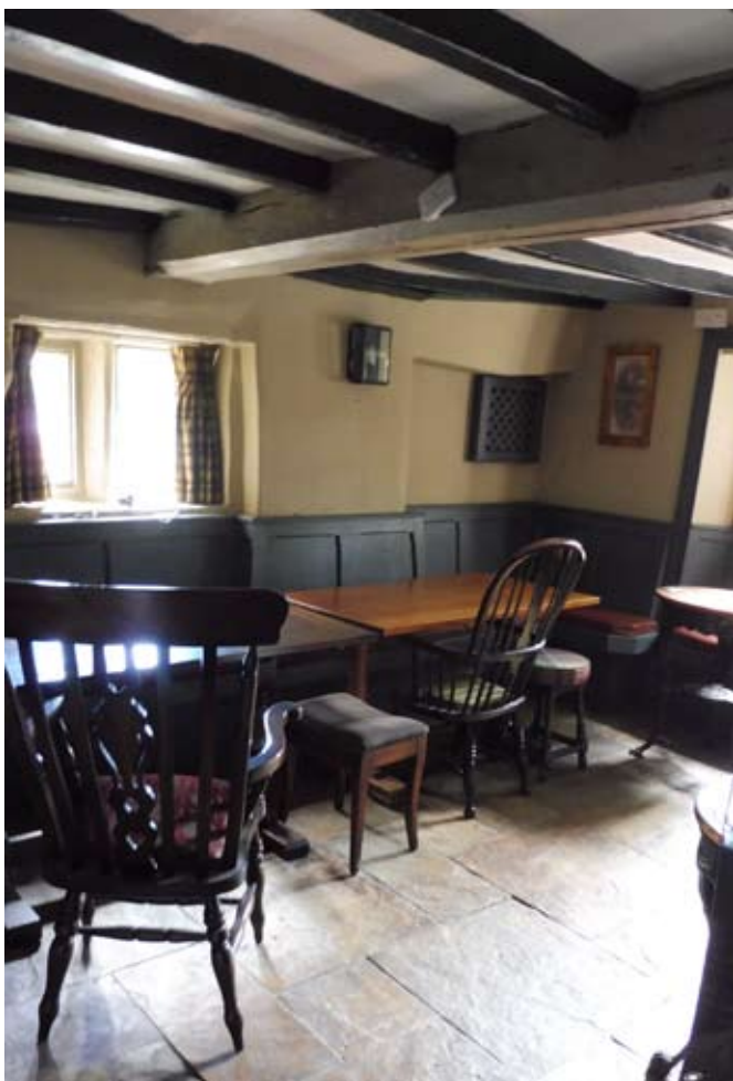
C17th Ground Floor - former doorway to RHS
