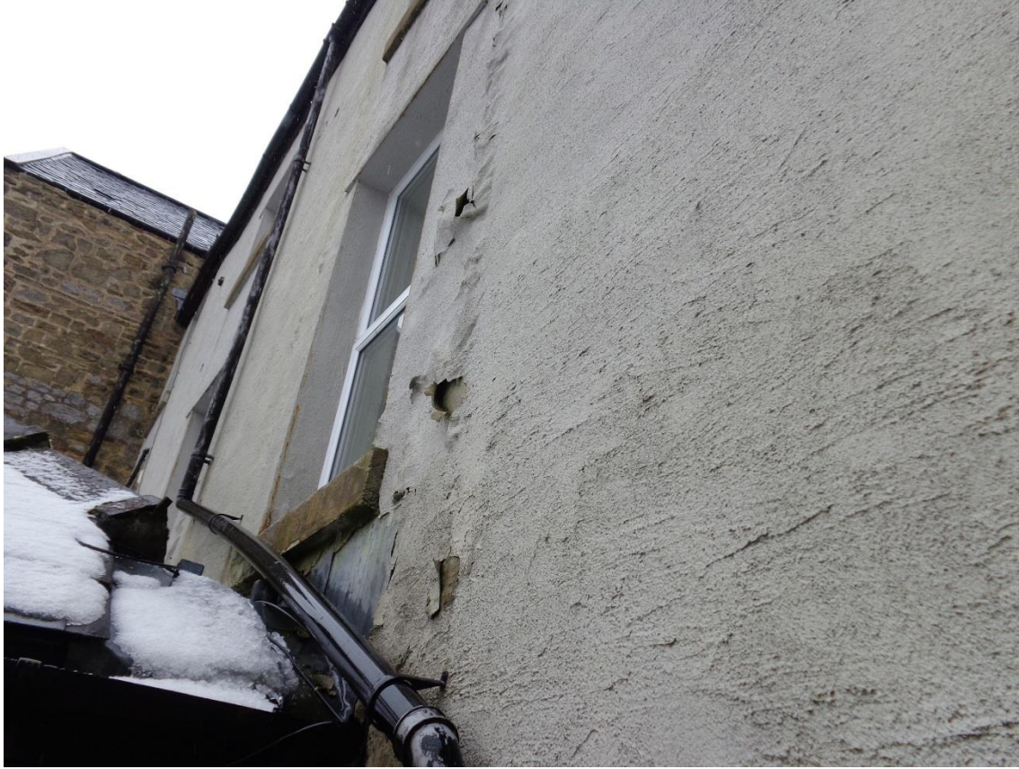
Photo 4 – Rear render to be replaced with breathable render.
