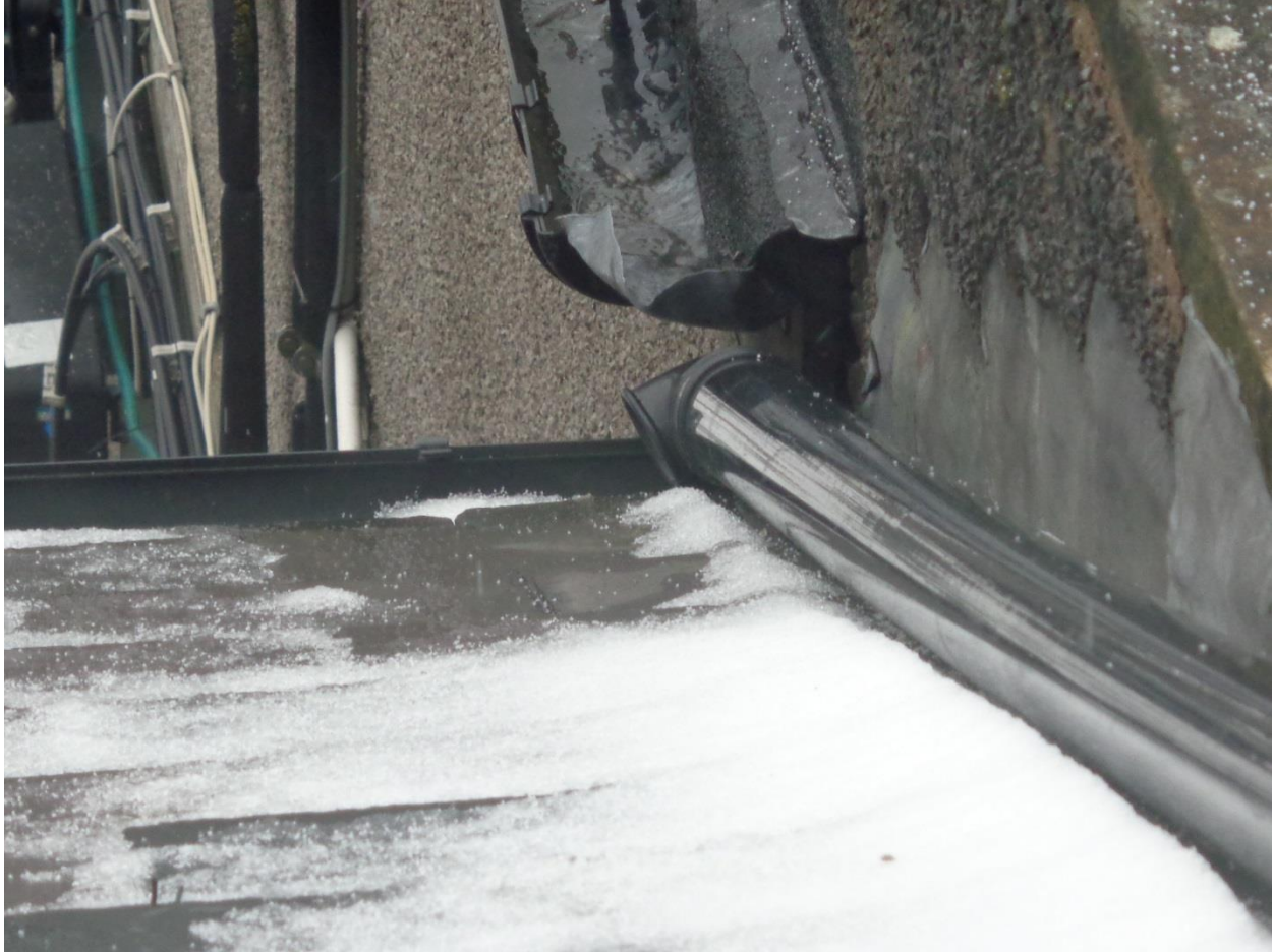
Photo 3- Existing Gutter system
