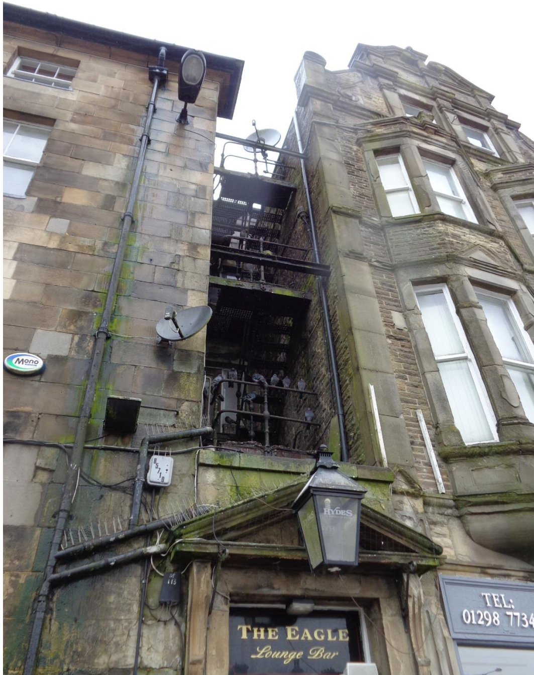
Photo 5 – Existing dilapidated fire escape to front elevation.
