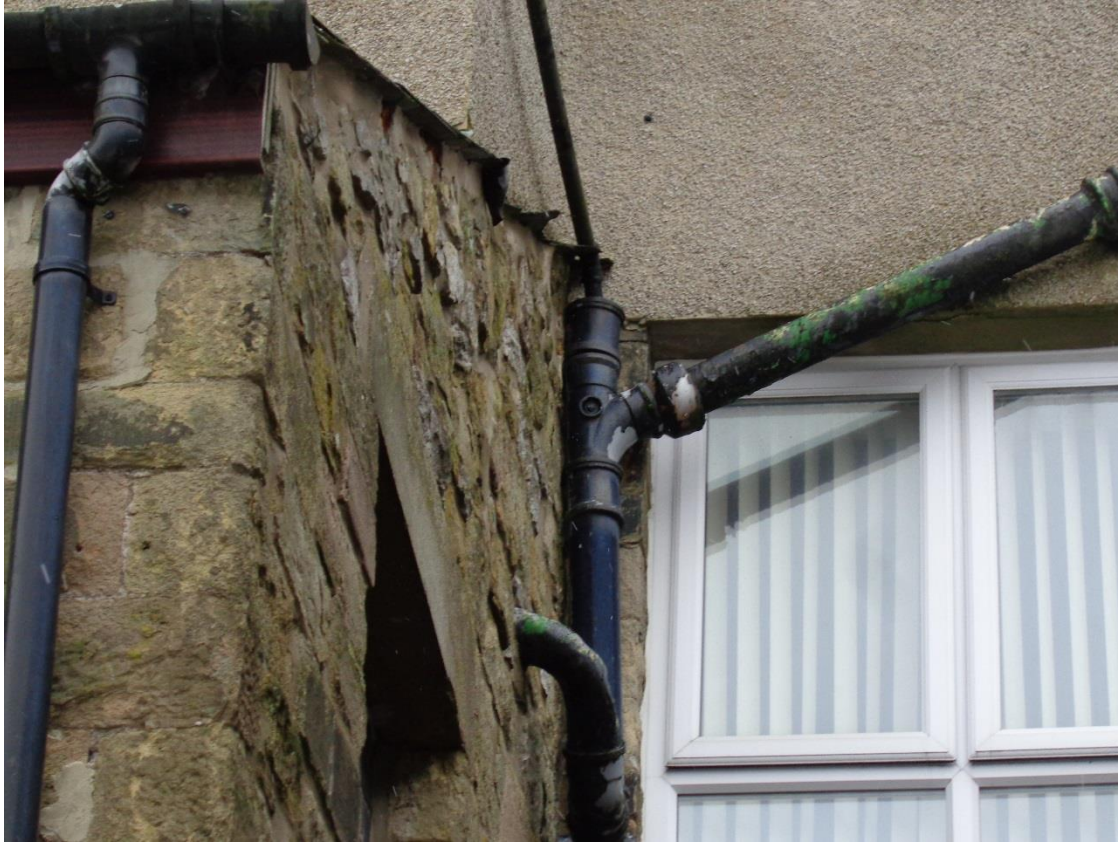
Photo 2 –Guttering to be replaced, impeding on window.
