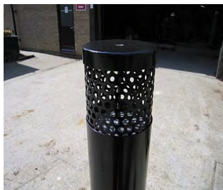
Example of Gas Vent
