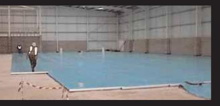
practice. When used in accordance with the manufacturer's instructions there will be no adverse effect on the membranes from underfloor heating under normal conditions of use, Alderprufe GRA will provide an effective barrier to the transmission of gases, liquid water and water vapour for the life of the concrete slab in which it is installed.
