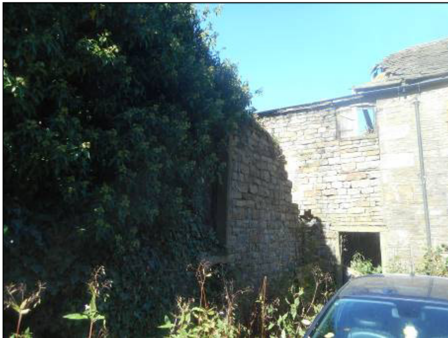
Photograph 1 - Southern aspect of building
