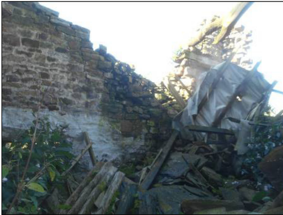
Photograph 3 - Internal view of building
