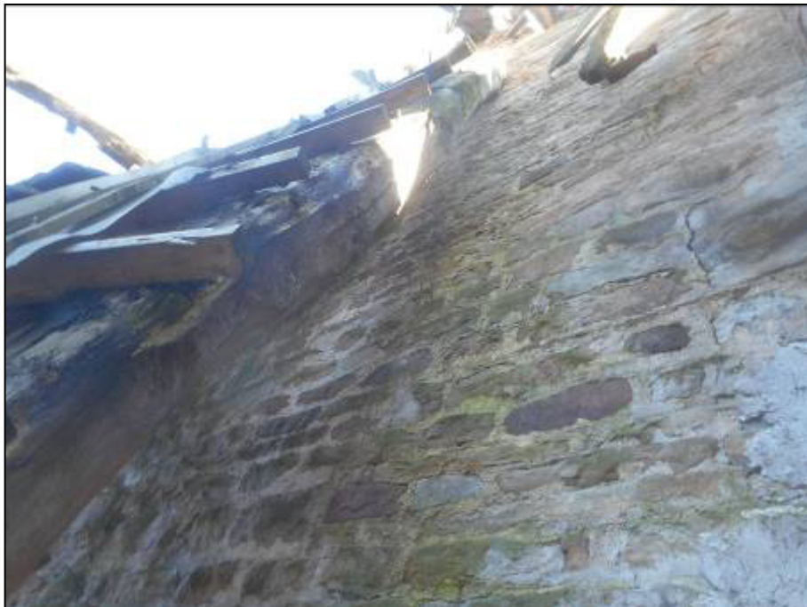
Photograph 4 - Internal eastern view showing gap to adjoining building now blocked
