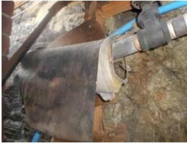
GE2 18 Bitumen to MMMF pipe
