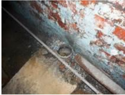
cement floor drain in concrete plinth
