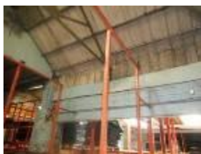
Corrugated AC between eaves and flat roof of F9B
