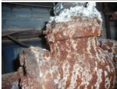
Sample GF4 07 Debris on valve F4 NADIS
