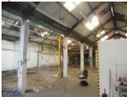
Non-asbestos insulation panels to roof and gables. AC gutter to base of rear gables. Presume ACMs to 2 Thermolier Space heaters
