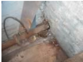
Cork insulation to pipework
