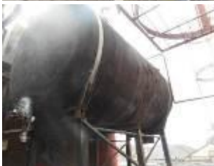
Sample GE2 15 Bitumen to MMMF insulation, tank E2
