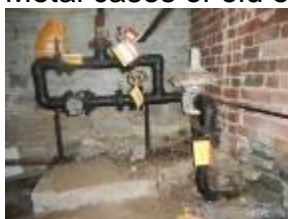
Gas supply pipework
