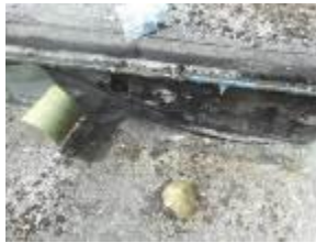
Sample GF5 09 Bitumen to roof upstand F5 NADIS
