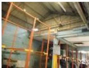
AC lining to internal face of roof and gables
