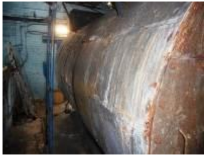
insulation behind metal sheets r/h side of boiler
