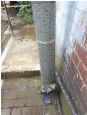
MMM with a bitumen wrap
