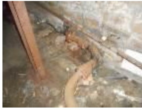
Un-lagged gas and water supply pipework
