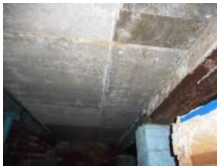
Poured concrete ceiling
