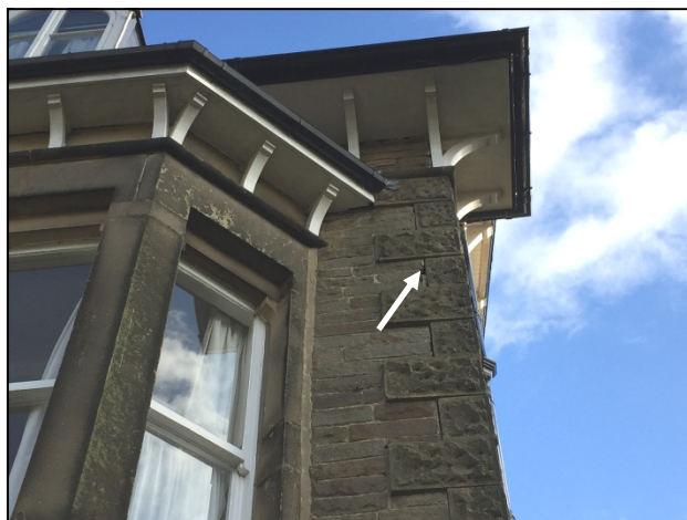
Plate 3 Gap where mortar has fallen away around quoins
