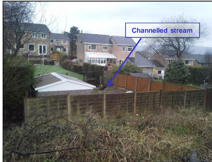
Photograph 5 – Stream channelled through rear gardens beyond western site boundary
