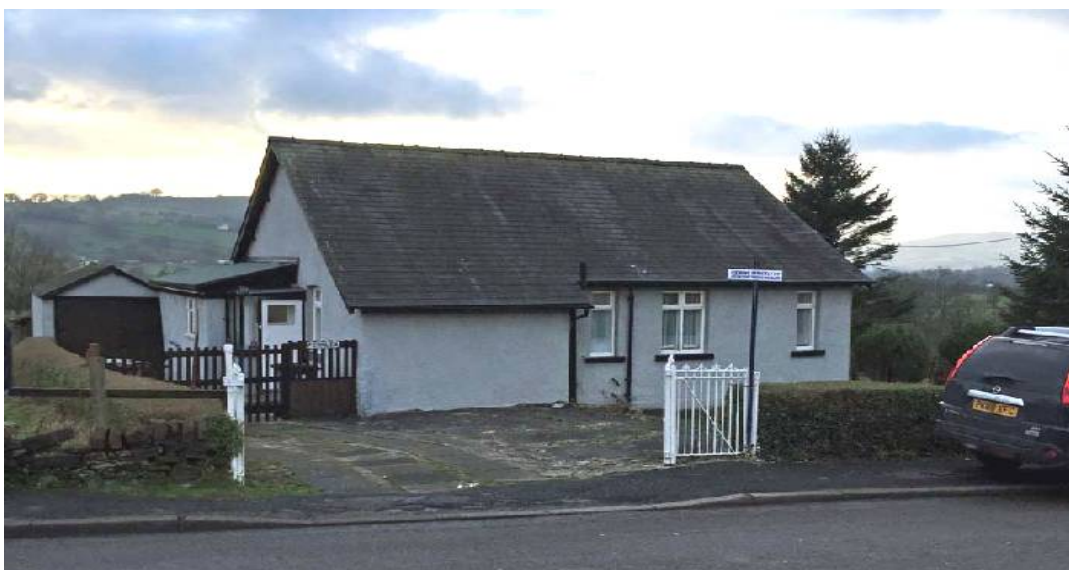
Fernlea outbuildings and entrance set well back from Buxton Road
