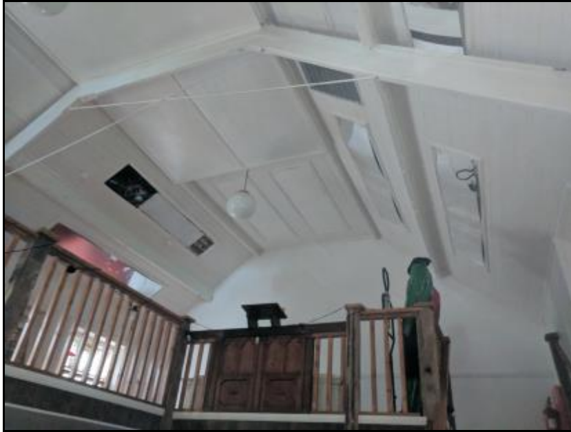
Photograph 8 showing the interior of the rear extension
