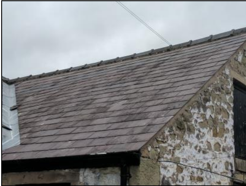
Photograph 10 showing the roof of the shippon
