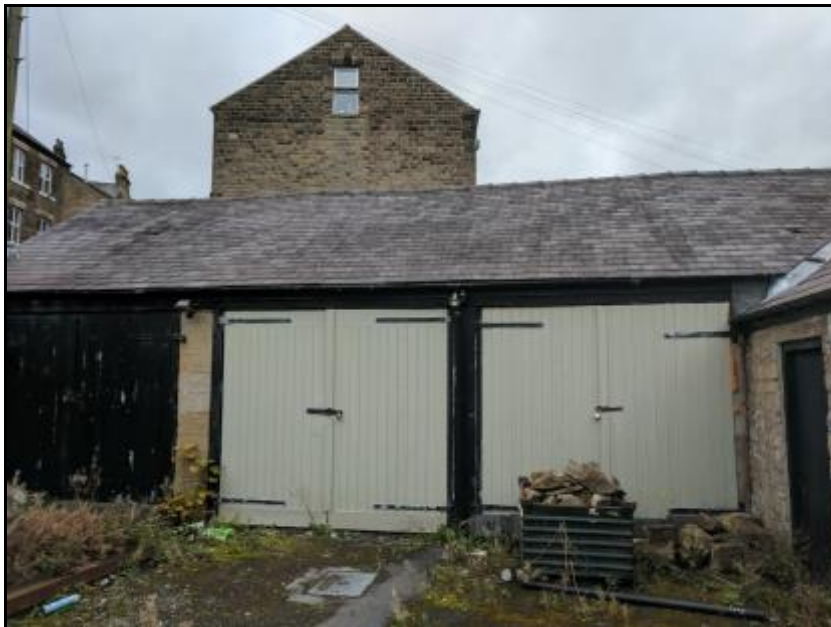
Photograph 11 showing the exterior of the garages
