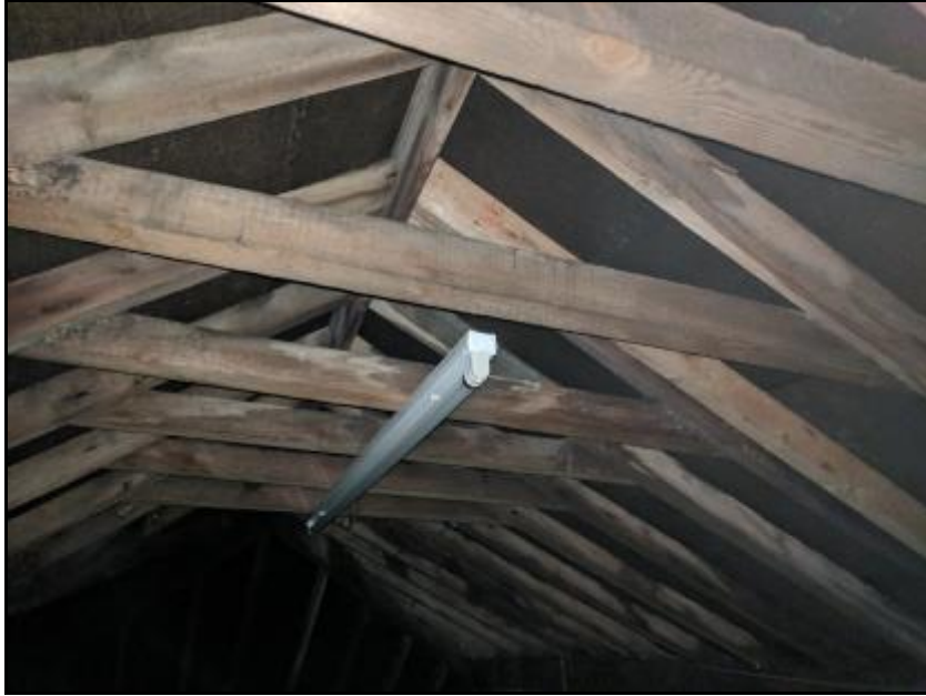
Photograph 12 showing the roof void of the shippon
