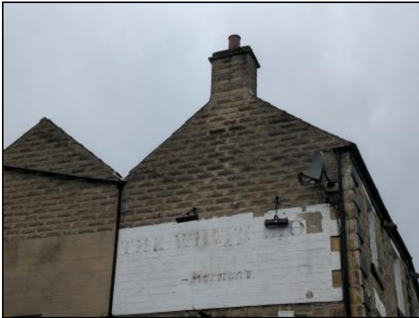
Photograph 1 showing the side elevation of the property
