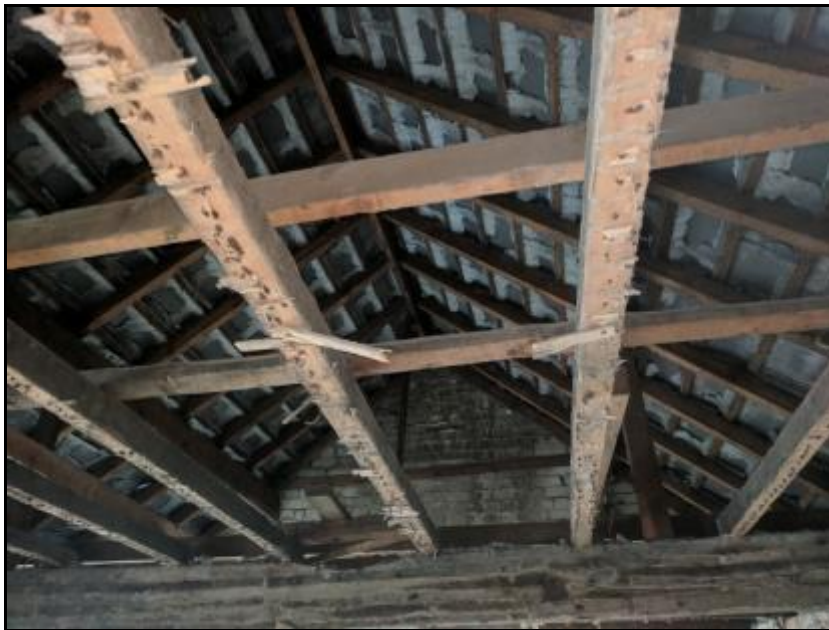
Photograph 7 showing the upper floors with removed ceilings
