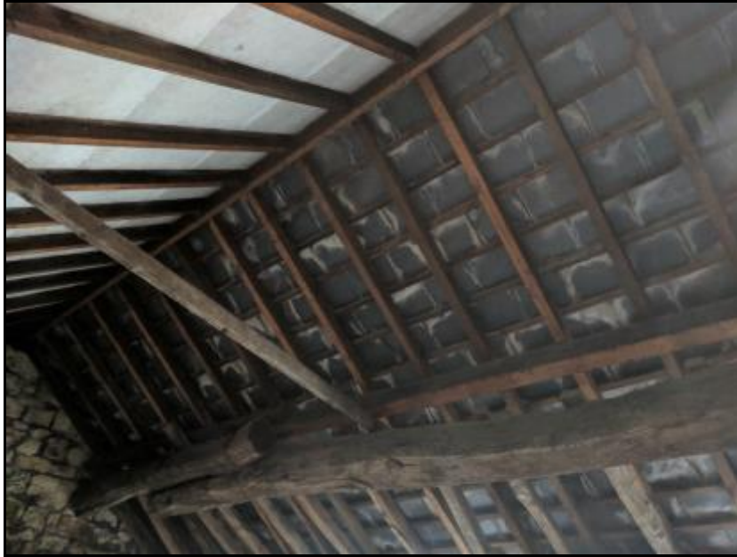
Photograph 6 showing the timber beams in the roof void
