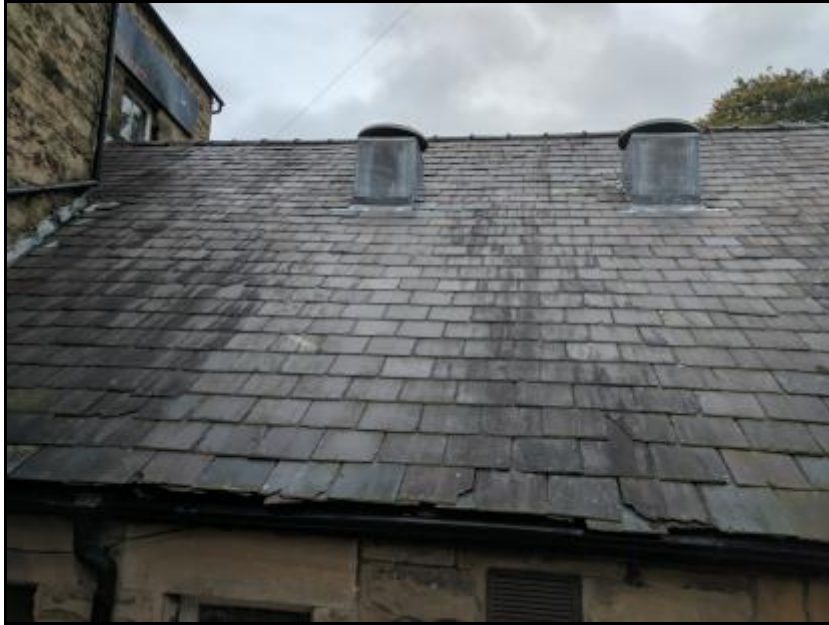
Photograph 4 showing the roof of the attached rear extension
