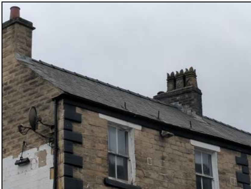
Photograph 3 showing the roof of the former public house
