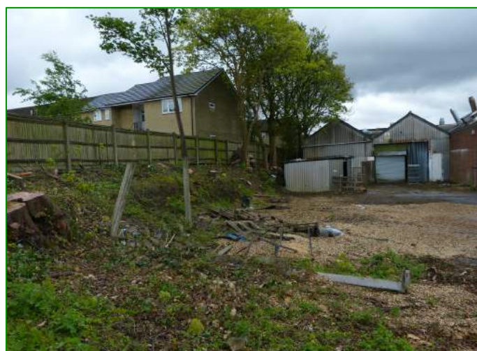
The east boundary, looking south
