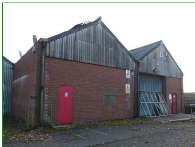
The north elevation of Building 2
