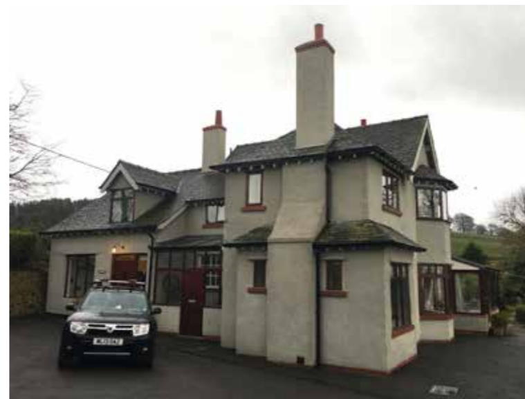
Side view to the front door from the west of the property
