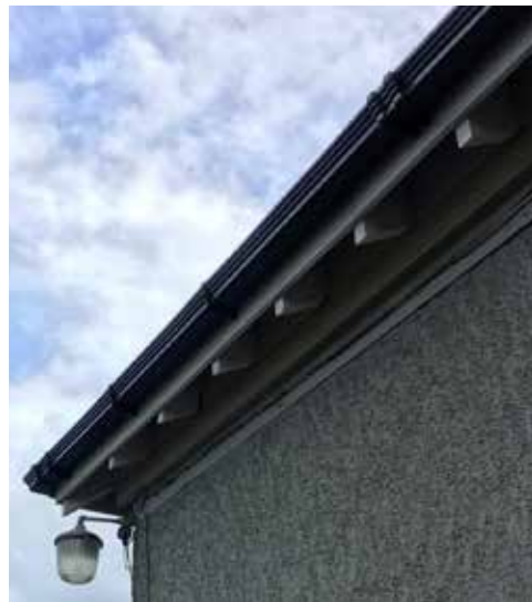
Image of existing projecting rafters to be replicated:
