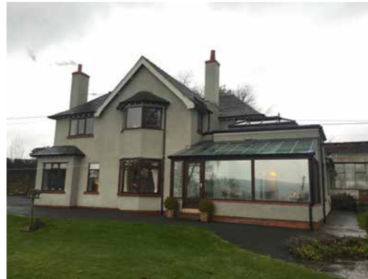
Front southern facade of property
