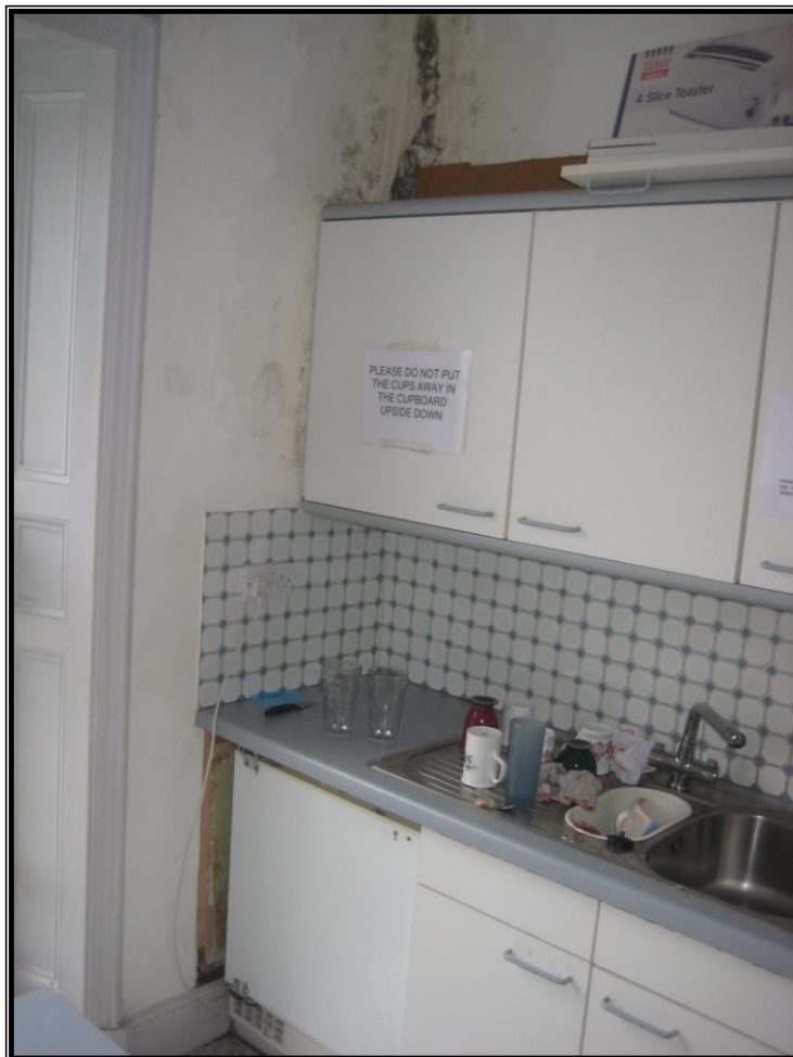
Figure 12: Kitchen at First Floor
