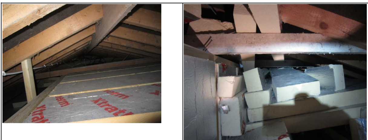
Photograph 9: View north from southern gable end
