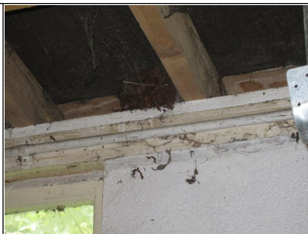
Photograph 10: Access at eaves of western elevation – note bird nest
