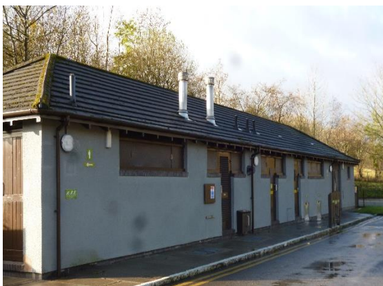
Plate 1. The toilet block with hipped clay tiled roof, grey rendering and chimney flues
