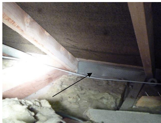
Plate 6. Bitumen felt lining with wire mesh at eaves.
