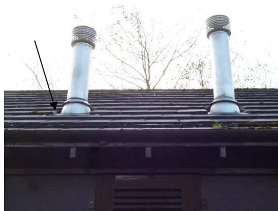
Plate 2. Gaps around base of chimney flues
