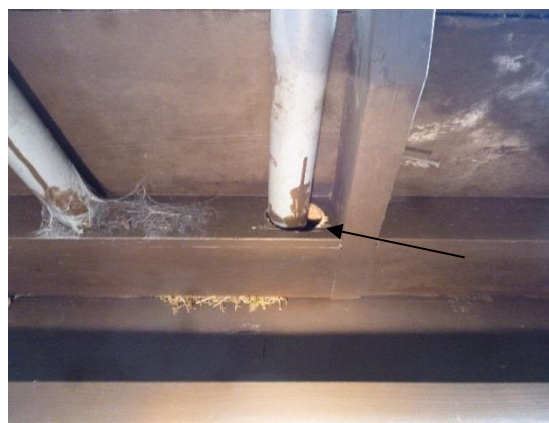
Plate 4. Gaps around pipe work as it leaves the roof at the eaves
