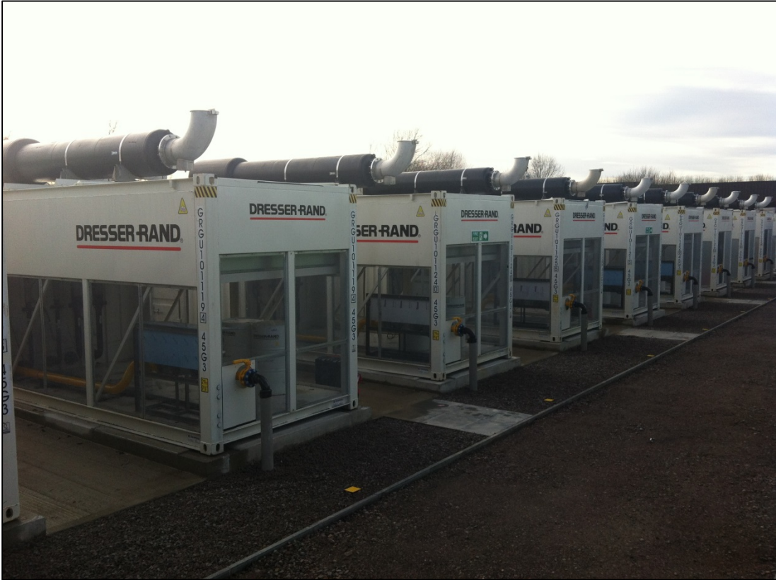
Figure 5 Typical Containerized generator
