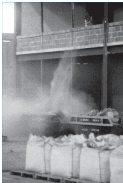
Figure 2.5 Material dropped into skips (Source: BRE Archive)
