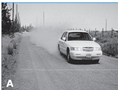
Figure 2.2 Road surface (A) without dust control and (B) with dust control (Source: www.brooksnsw.com.au )
