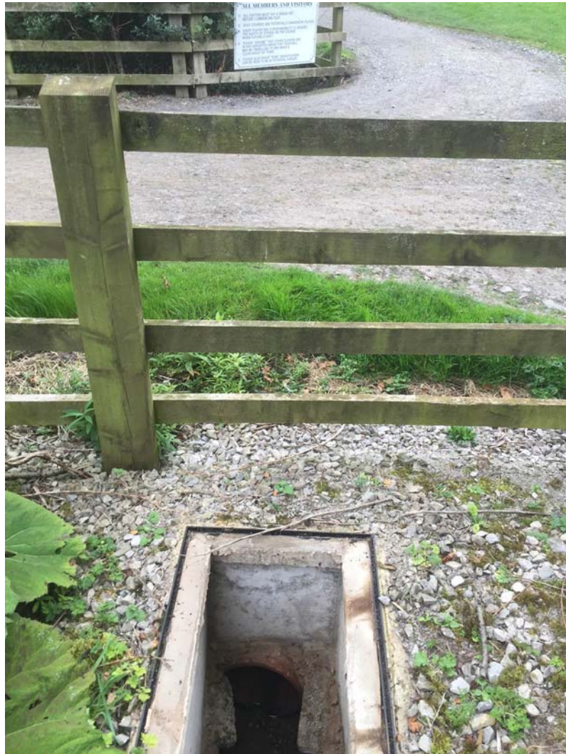
Photo 10 – 225mm pipe from ditch under access road and into manhole.
