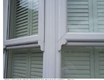
REPLACEMENT UPVC WINDOW TO REAR ELEVATION - 70MM CASEMENT WINDOW WITH SASH HORNS NO GLAZING BAR TIMBER SASH REPLACEMENT TO FRONT ELEVATION COMPOSITE DOORS TO BE UTILIZED TO BOTH ELEVATIONS
