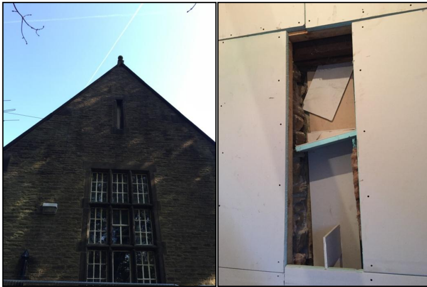
Figure 6. Boarded ventilation gaps within main building.
