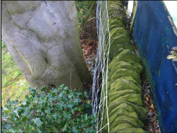
Image 3 – Close up view of the drop in level adjacent to Tree 4
