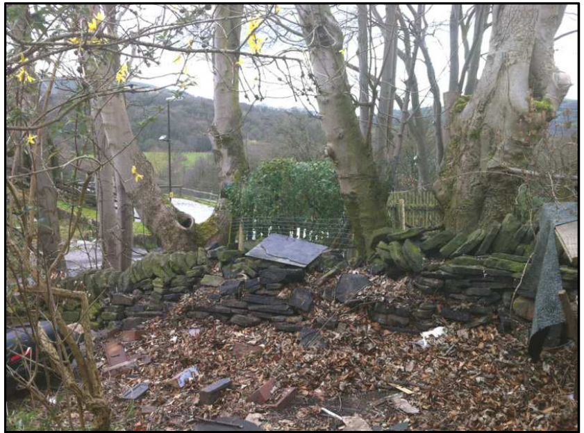
Image 7 – View looking South at Trees 1 [Left] 2 and 3 behind the stone boundary wall
