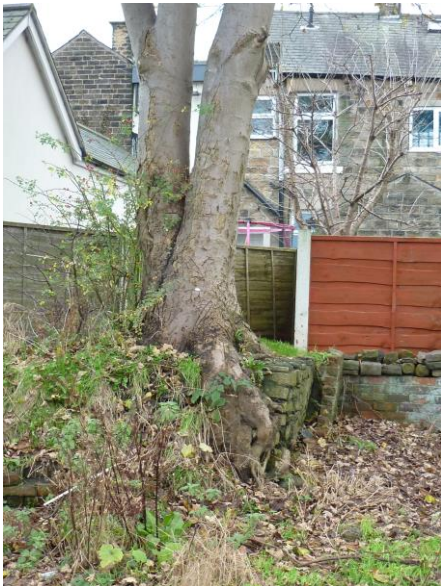
450 Sycamore showing exposed roots, subsiding wall and concrete surface
