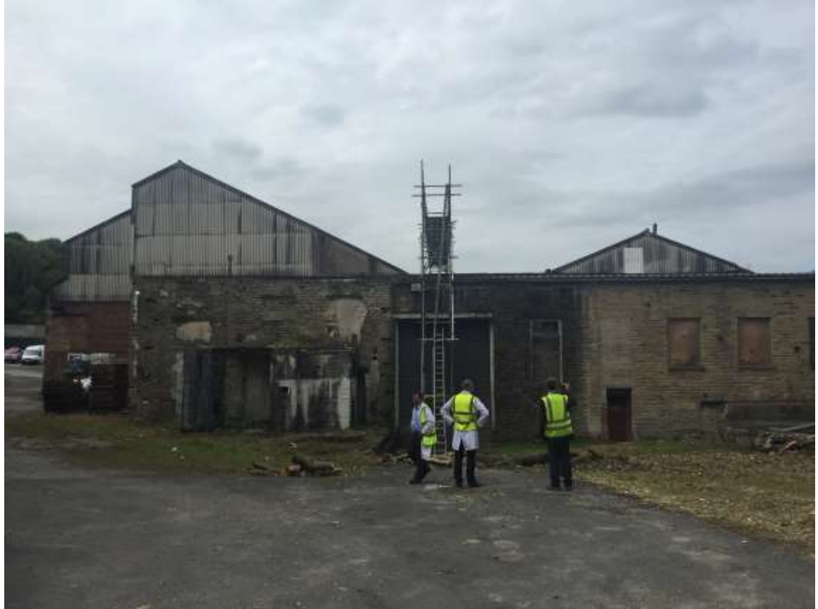
East end of the mill showing lean-to stone building and high asbestos clad roof.
