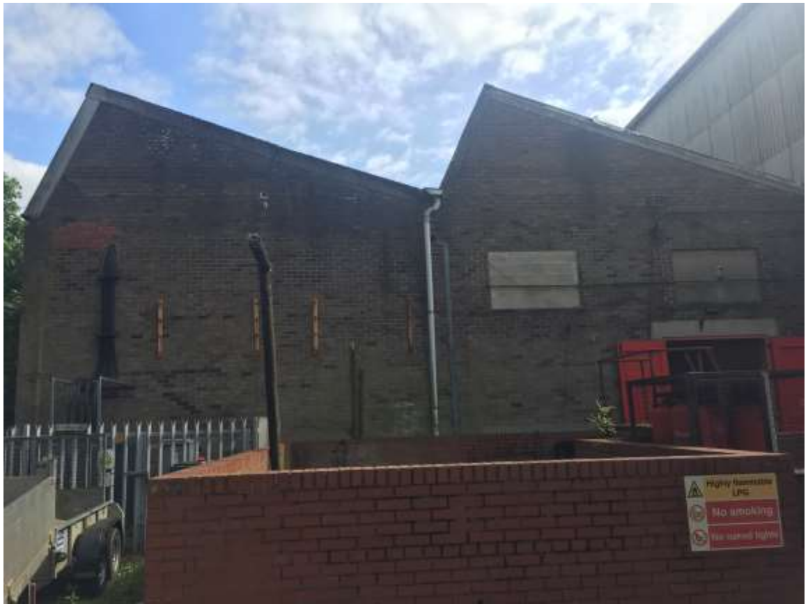
West end of the mill showing north light roof
