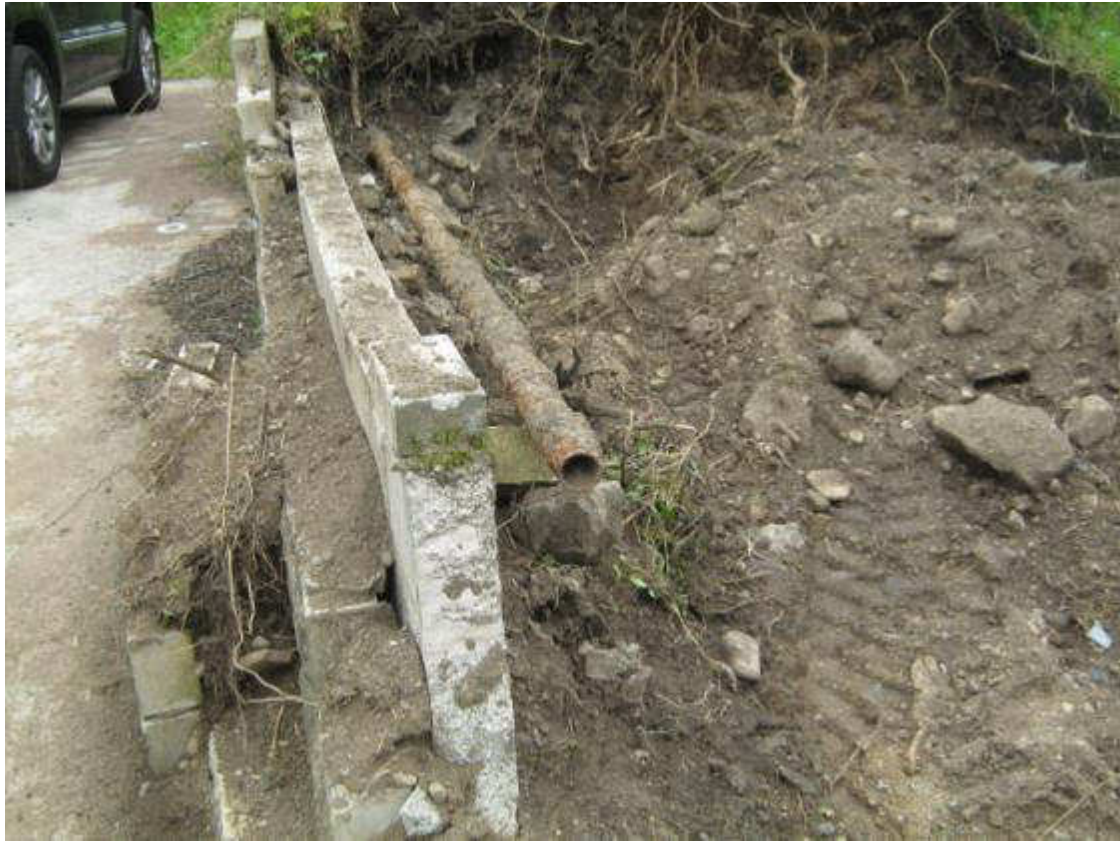
Photo 15: Damaged wall and disconnected pipework
