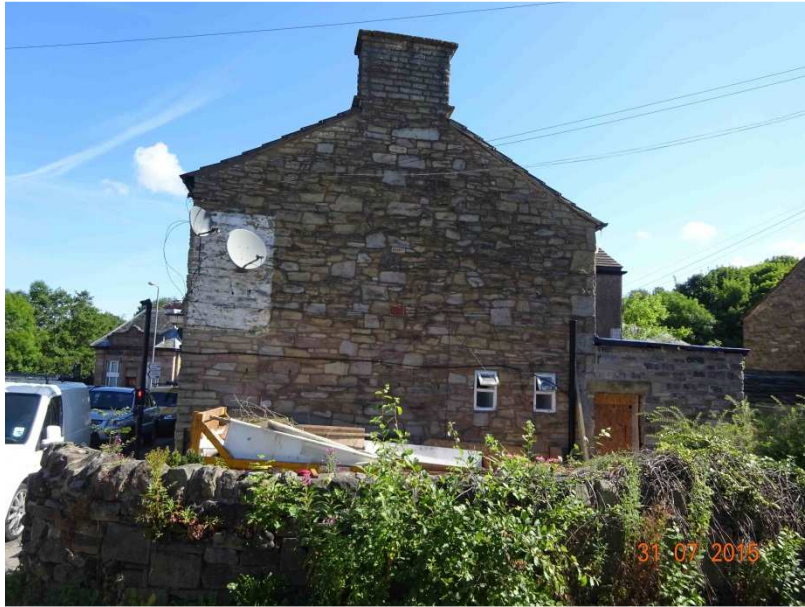
Photo showing side of 110 Buxton Road
