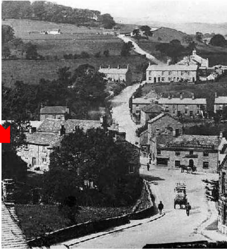
Rear view prior to rear extensions being built
