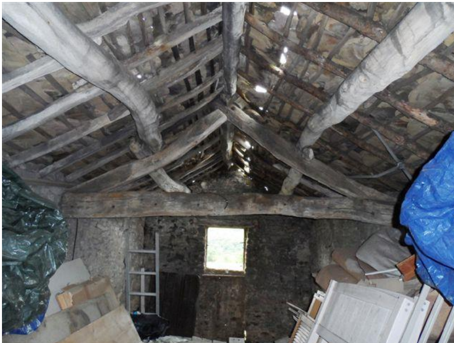
Internal barn showing open roof
