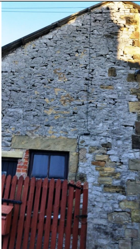
Plate 3 – View of far west side of building with extending gaps in stonework
