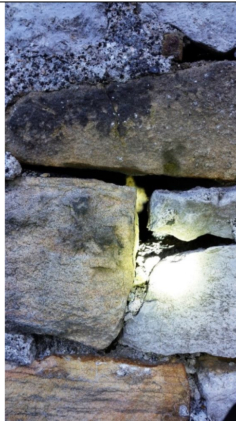
Plate 4 – Close up example of extending gaps
