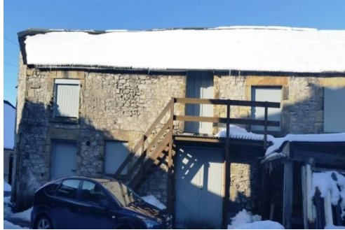
Plate 3 – View of far west side of building with extending gaps in stonework
