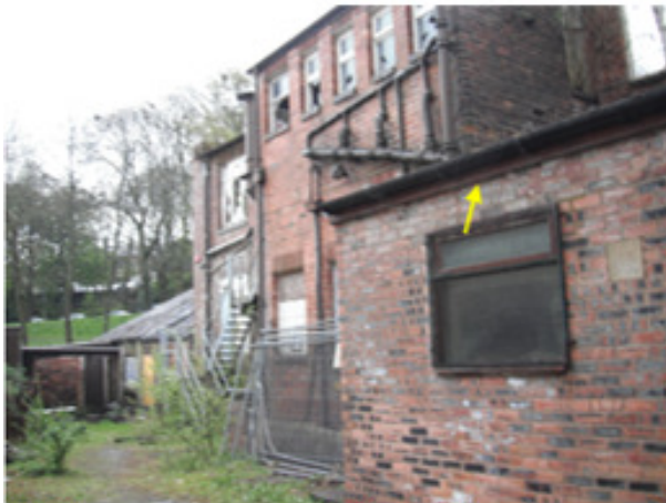
P3 N. aspect, gaps under barge boards
