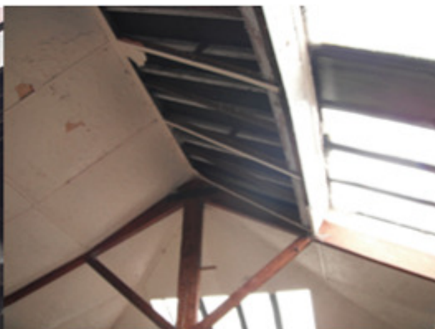
P8 Building 2, board-lined slate and skylights
