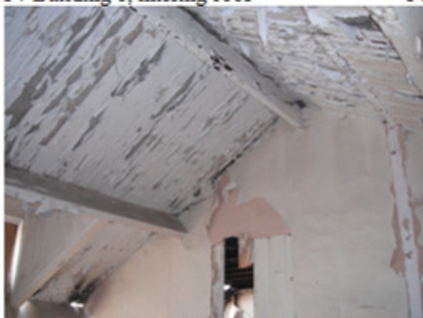
P9 Building 4, board-lined slates, some slates missing.
