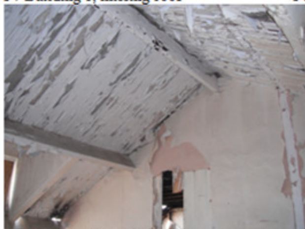
P9 Building 4, board-lined slates, some slates missing.
