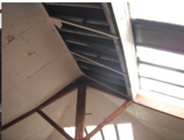
P8 Building 2, board-lined slate and skylights
