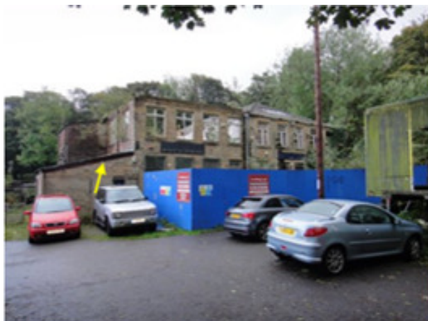
P1 NW aspect, gaps under barge boards
