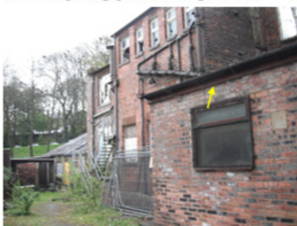
P3 N. aspect, gaps under barge boards
