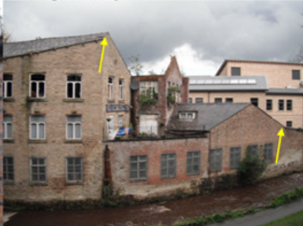
P4 S. aspect, gaps under roofing slates
